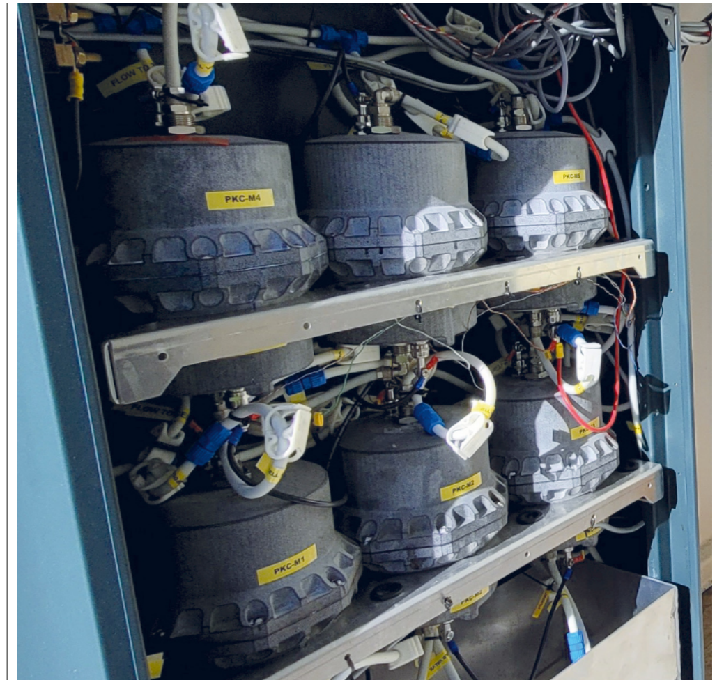
SLIQ flow cells made of high density polyethylene and with 100% reusable catholyte. (Picture courtesy of StorTera)
