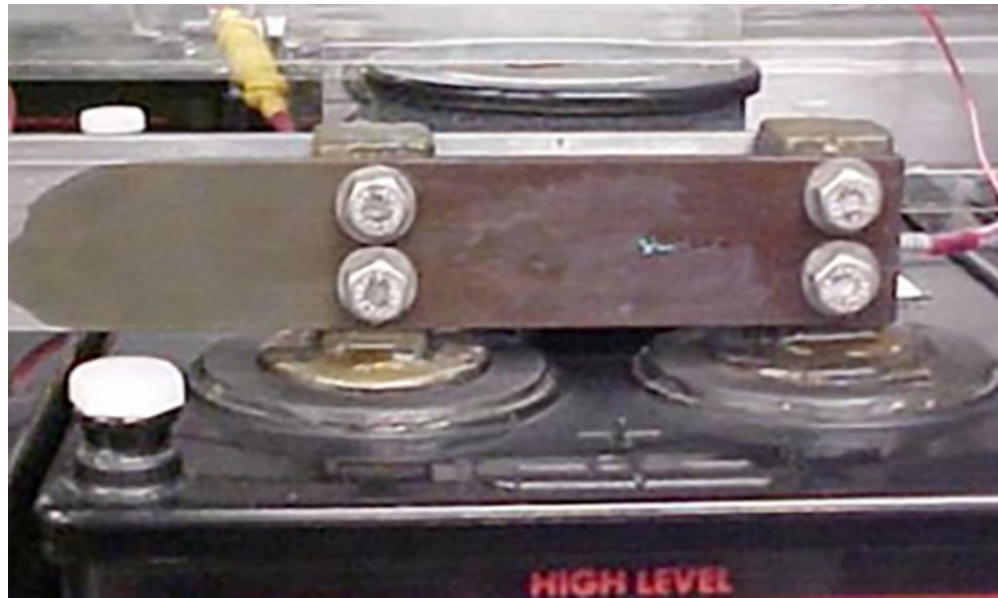
Fig 6: Moderate terminal lead peroxidation (brown colour) on the right-most terminal extending to the left resulting from a post seal leak.
